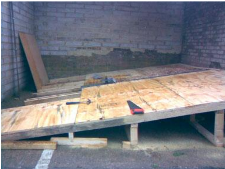
Sloping floor of the wood chip store
